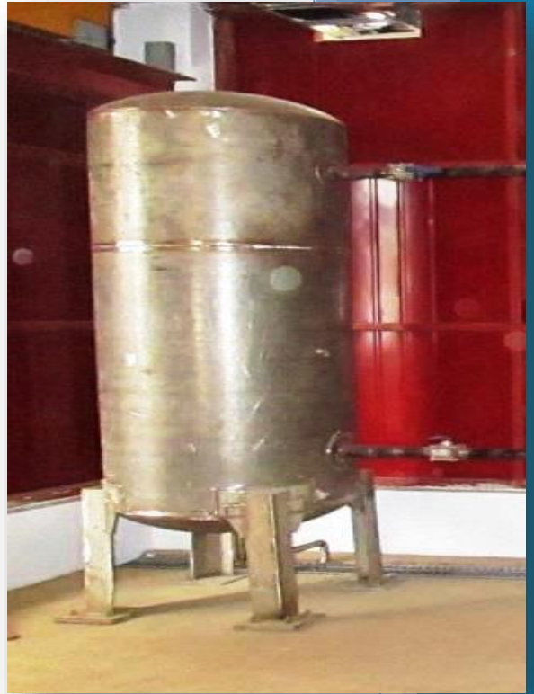
COMPRESS AIR TANK
