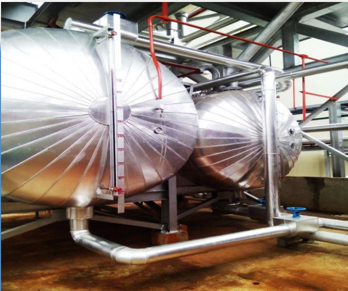
INSULATION AND CLADDING WORKS FOR LFO AND HFO TANKS
