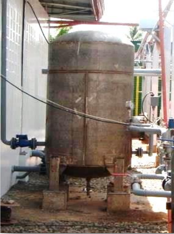
RAW WATER PRESSURE TANK
