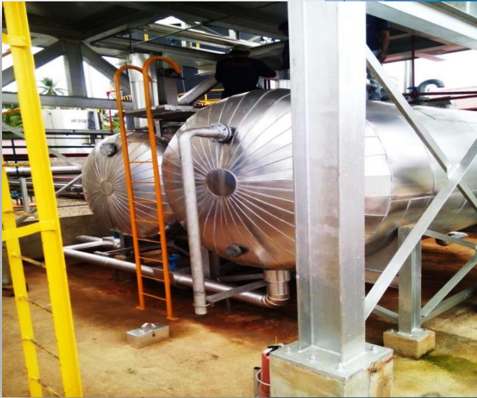
INSULATION AND CLADDING WORKS FOR LFO AND HFO TANKS
