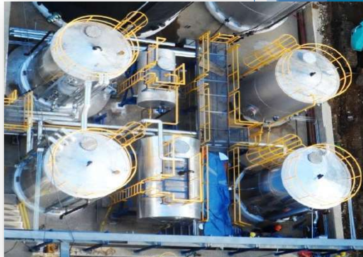
INSULATION AND CLADDING WORKS
