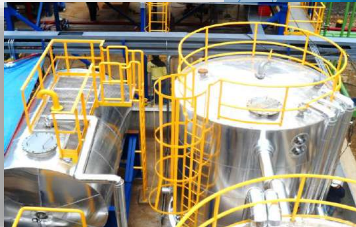
INSULATION AND CLADDING WORKS
