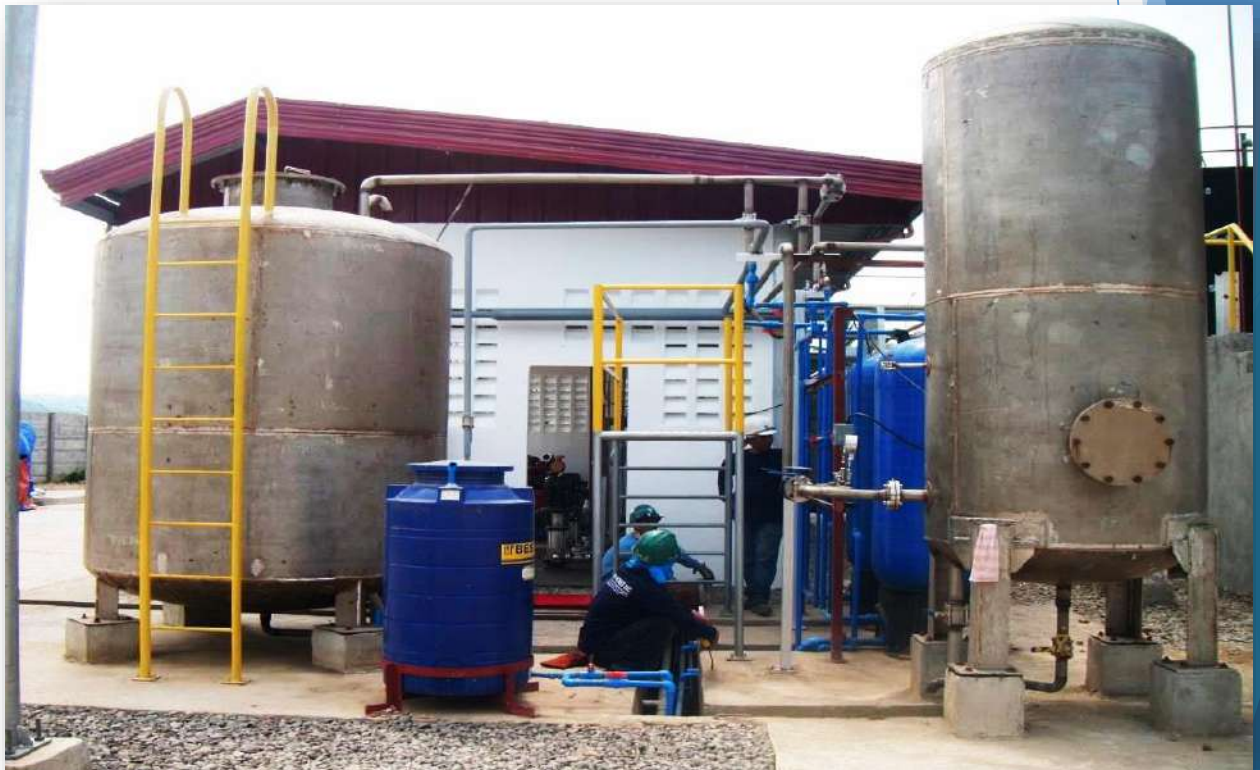
SOFTWATER STORAGE TANKS
